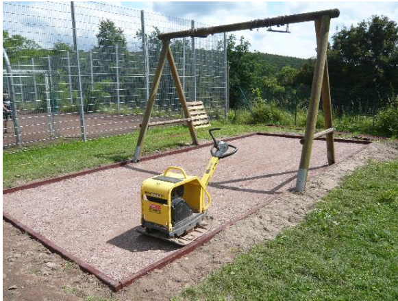
Crushed stones bed stable compacted
