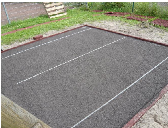
Leveling crushed sand/stone chippings
